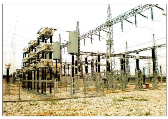
((Capacitor Bank 150kV 25Mvar - GI Duri substation in Indonesia))
