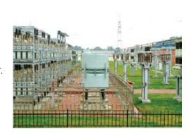
Therefore, SVC is mainly installed near high and rapidly varying loads, such as arc furnaces, chemical plants where need to smooth flicker voltage.
