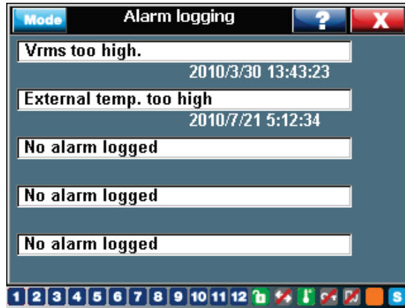
Figure 50: Bank monitoring alarm logging
